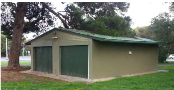
Existing Maintenance Shed
