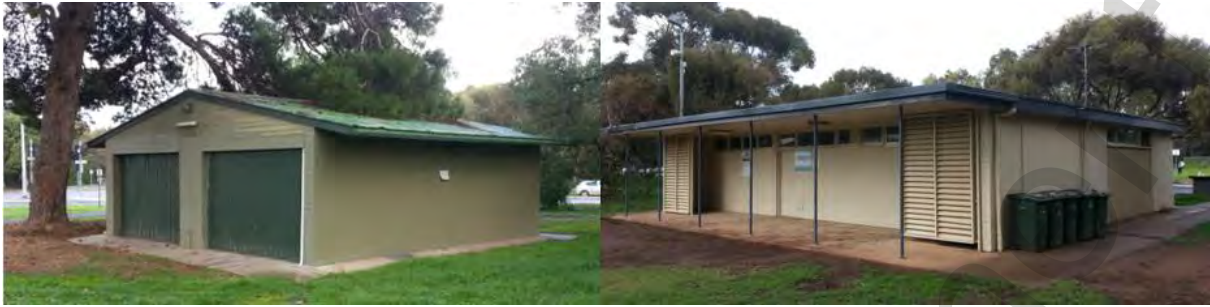
Existing Buildings in Park 9
