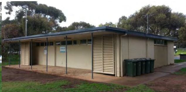
Existing Changerooms with Public Amenities at the rear
